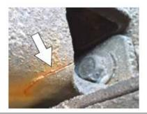
No cracks are permitted. No welding or other repairs are permitted
